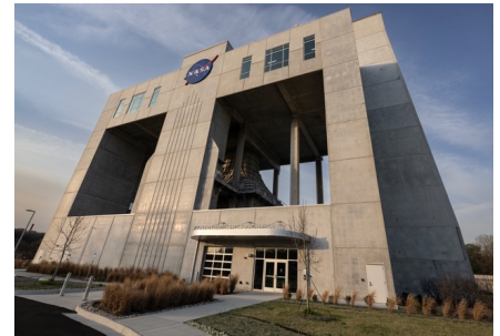
Fig. 8. FDRF building (note exposed contraction cone at center)
