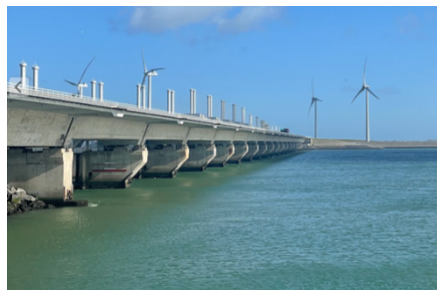
Section of the Delta Works
